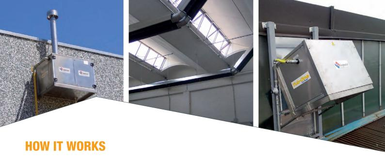
**TUB•ONE**® gas-fired radiant strips transmit heat by radiation, directly heating people and objects, resulting in an immediate thermal comfort without moving air. Heating takes place by means of an electromagnetic infrared waves propagation that transports thermal energy in a straight line, thus generating heating transmission.
